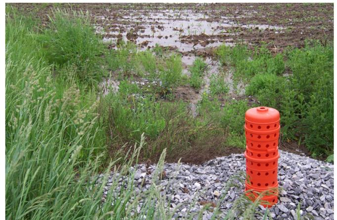
Standpipes (also known as surface inlets or tile risers) are vertically installed surface pipes placed at the low point of a field that are connected to and routed through an existing tile network. Standpipes allow surface water from a field to flow directly into a tile drainage network and out the outlet. In case of a tile blockage, standpipes can also release water to the surface.
